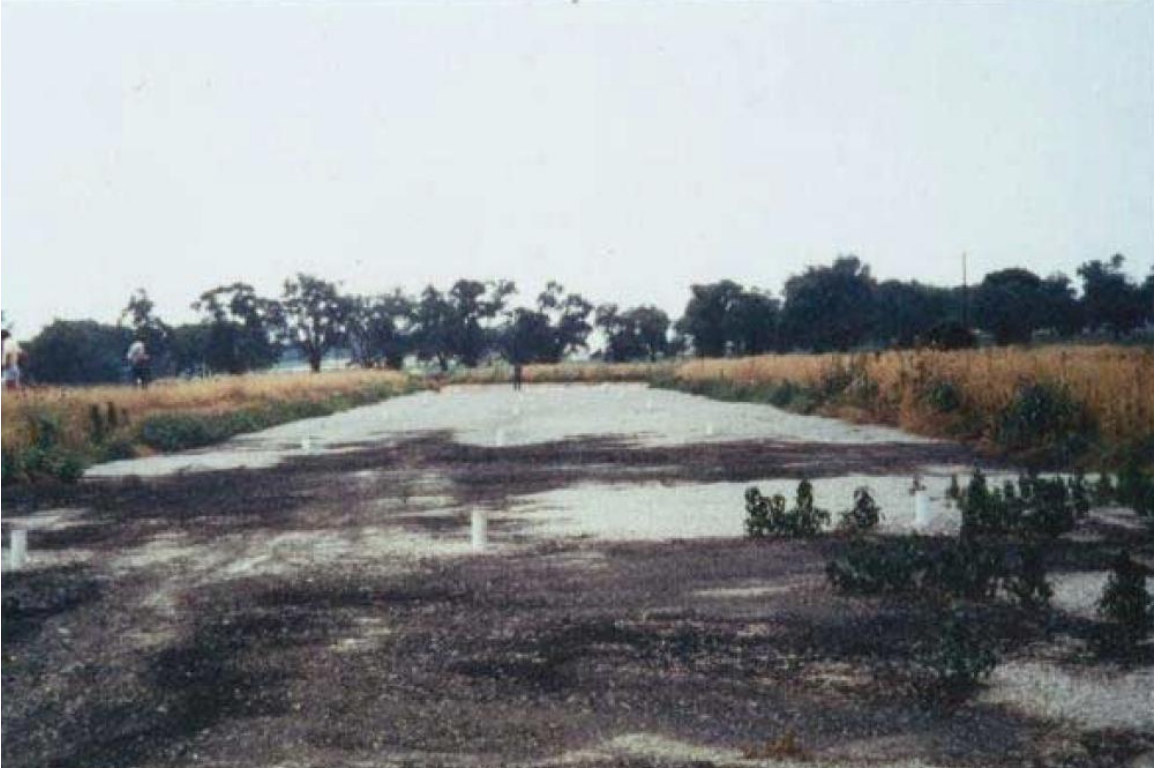
Sample photo of a subsurface flow system under construction
