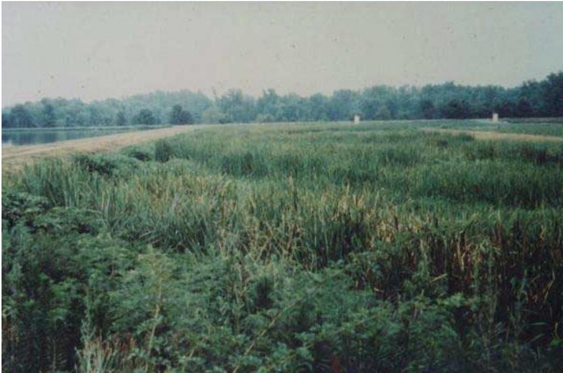
Sample photo of a subsurface flow system completed
