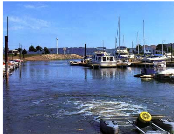
Triton O2 propeller type aerator in operation in a typical lagoon
