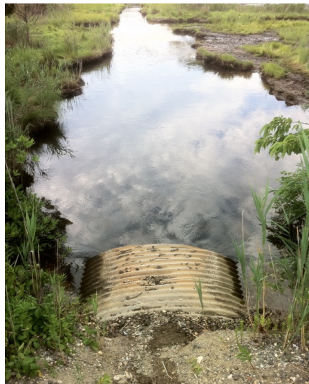
Intake pipe sending purified water from the salt marsh back to the lagoon between Bayview Ave. and Amherst Drive 400 east of Veeder Lane
