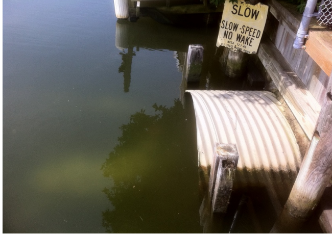
48" Outfall pipe at 102 Moorage Ave. that carries most of the effluent from the 160 acres to the west of Berkeley Shores
