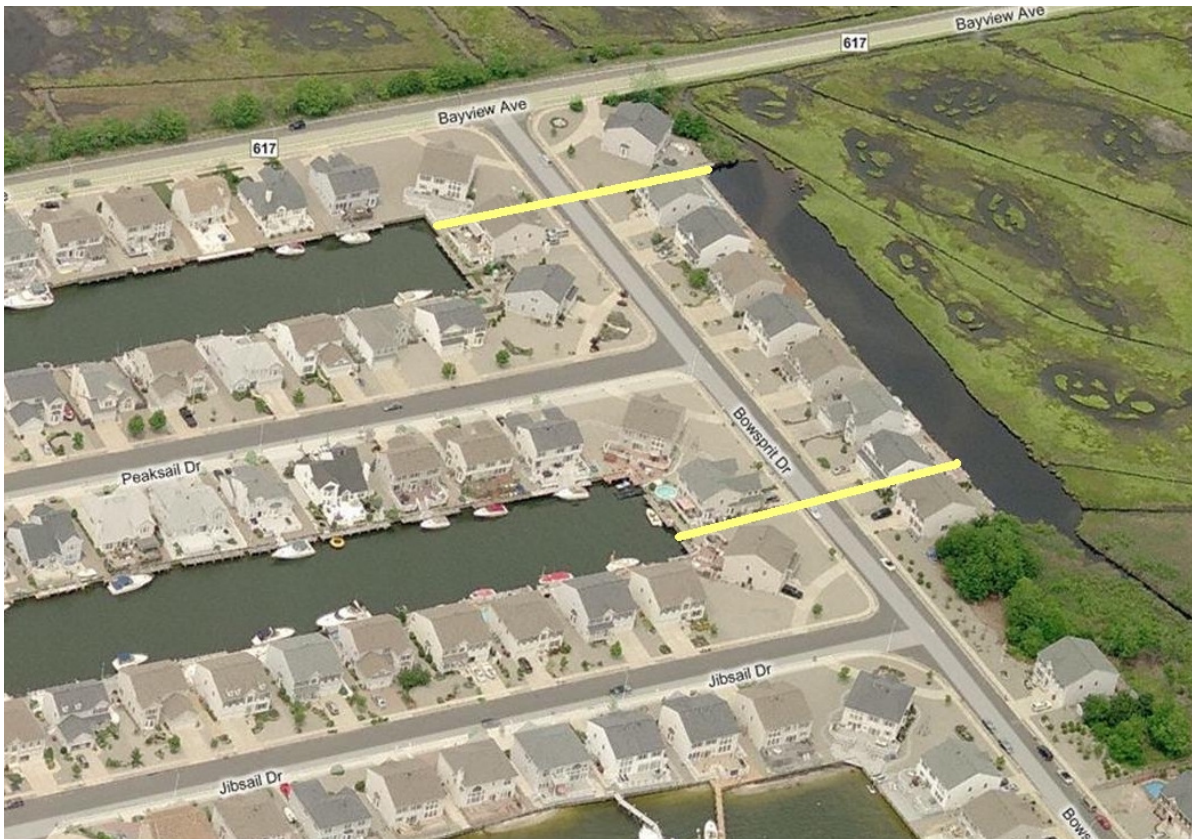
Another possible location for a tidal circulation pipe is between the lagoon ends on the west side of Bowsprit Drive and 46 acre salt marsh on the east side of Bowsprit Drive. Notice the water quality color between the lagoons to the left and the salt marsh lagoon.
