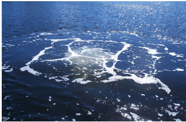
Bubbles from an air difuser resting on the bottom of a lagoon
